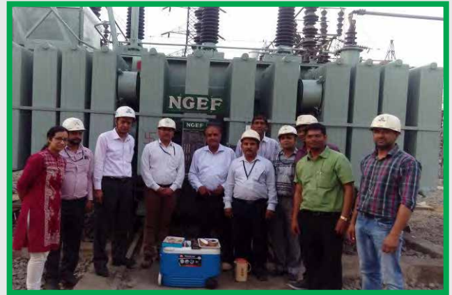
26.5 MVA 132KV Transformer overhauling at M/s NFL, Panipat
